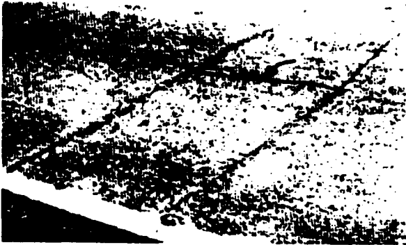
Fig. 3.2.4.8(a) — Punchout, Severity 2
